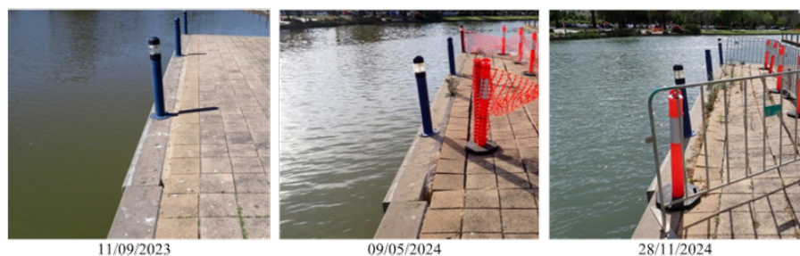
Figure 12- Progression of Section 4 Wall Toppling Failure
