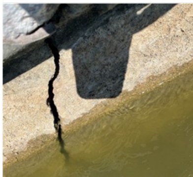
Figure 13- Cracks observed along upper perimeter of lake edge wall
