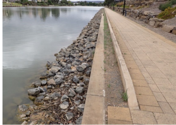
Figure 8- Delfin Lendlease Repair Works with Upright Kerbing
