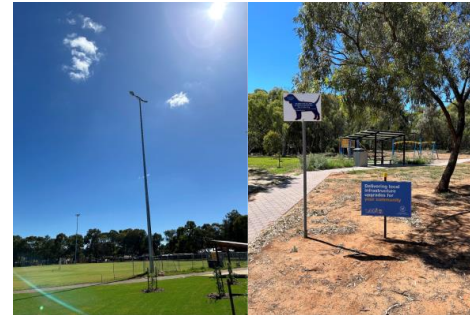
Sports lighting upgrade, Yalumba Drive Reserve, Paralowie
