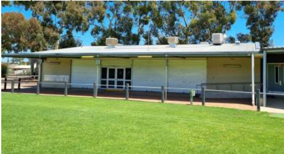
Salisbury Oval Roof & Veranda Replacement – Before Construction
