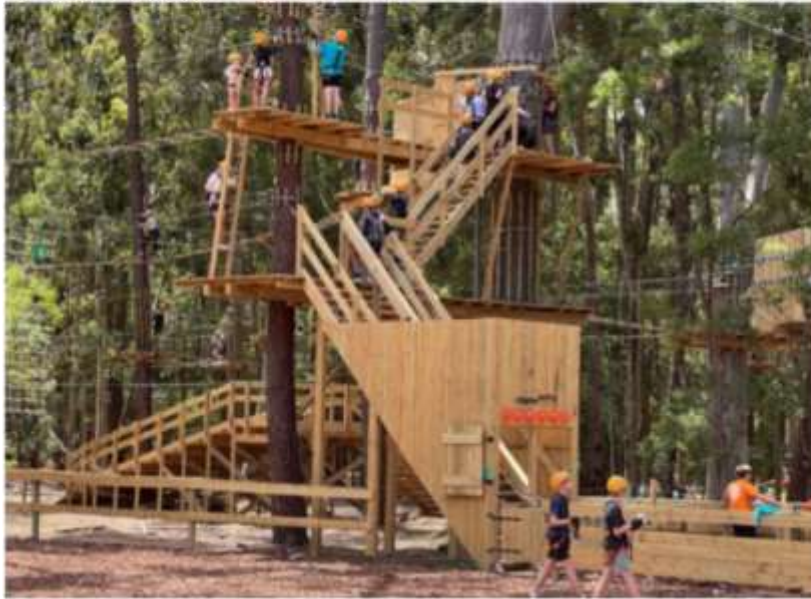
Figure 4-3 - Access Platform (Kuitpo Example)
