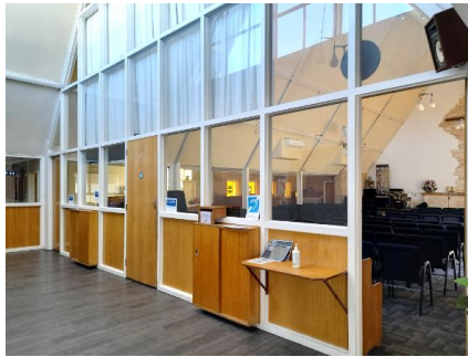
Glazed partition wall between foyer and chapel
