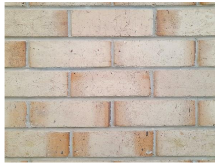
Face brick in chapel
