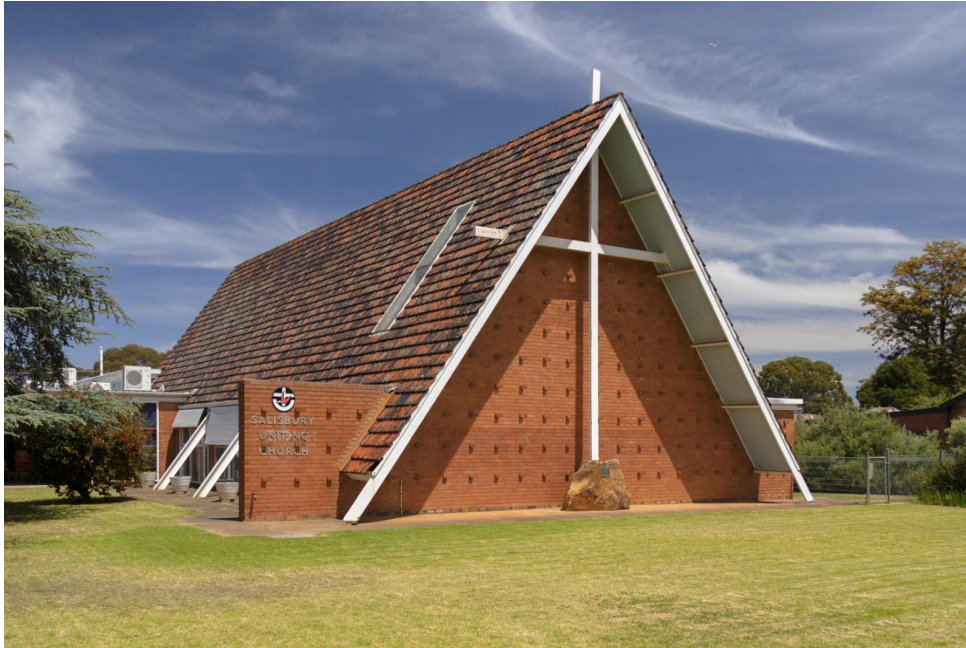
Former Salisbury Methodist Church, 2 November 2023
