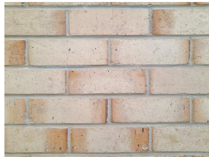
Face brick in chapel
