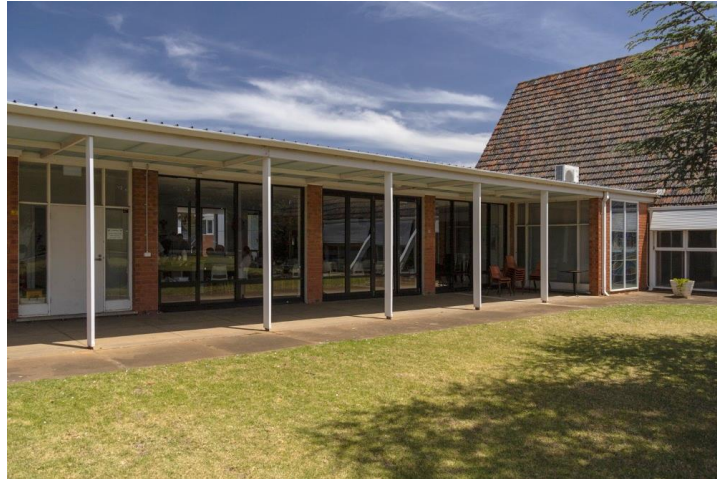
East wing showing verandah and new door openings
