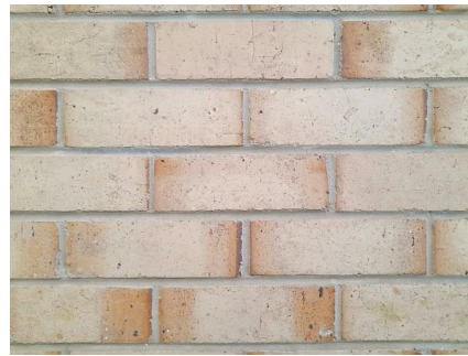
Face brick in chapel
