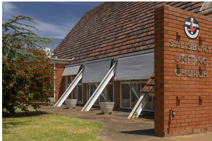
Eastern side showing A-frames and wing wall with sign (on right)
