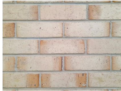
Face brick in chapel
