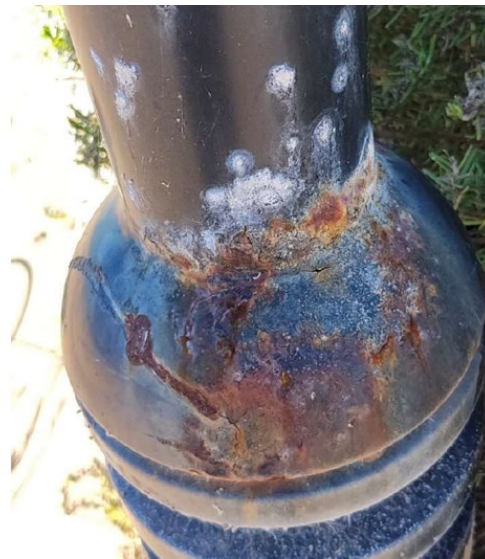
Figure 2. Light pole with moderate corrosion.
