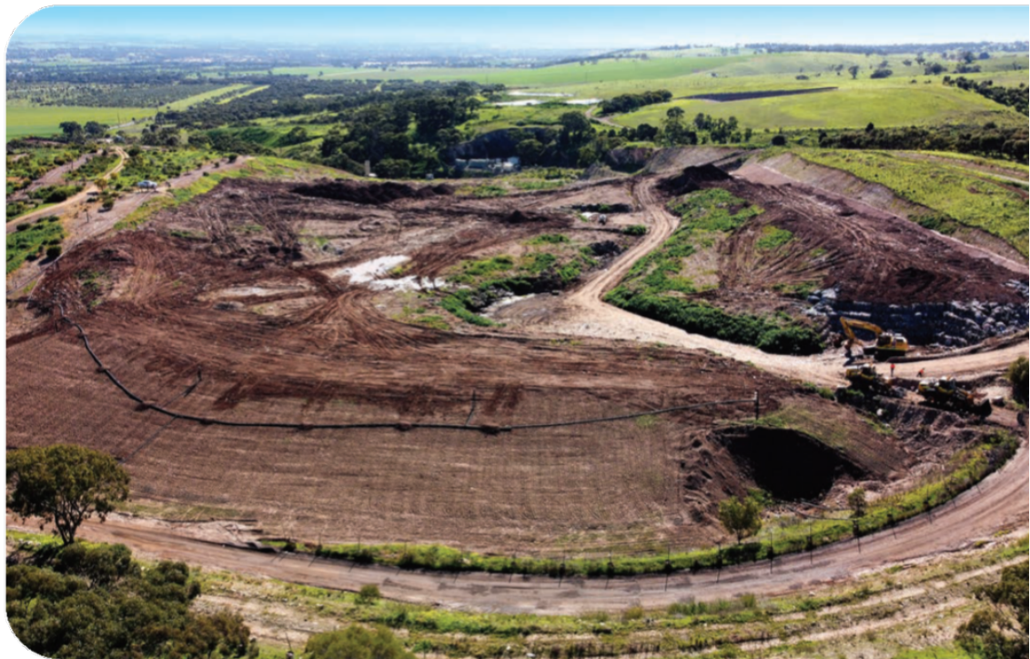
NAWMA's combined renewable energy facility generates over 8,468,401 kwh of electricity per year.
