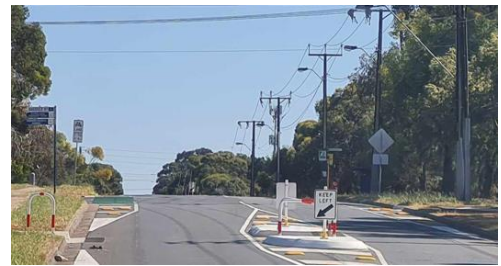
Pedestrian Refuge Nelson Road, Para Vista
