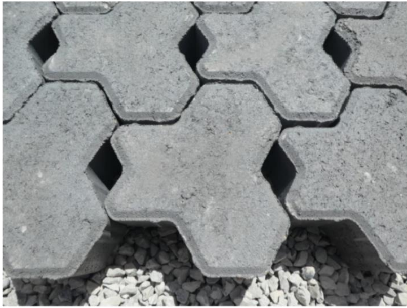
'Ecotrihex' pavers on washed aggregate drainage layer.
