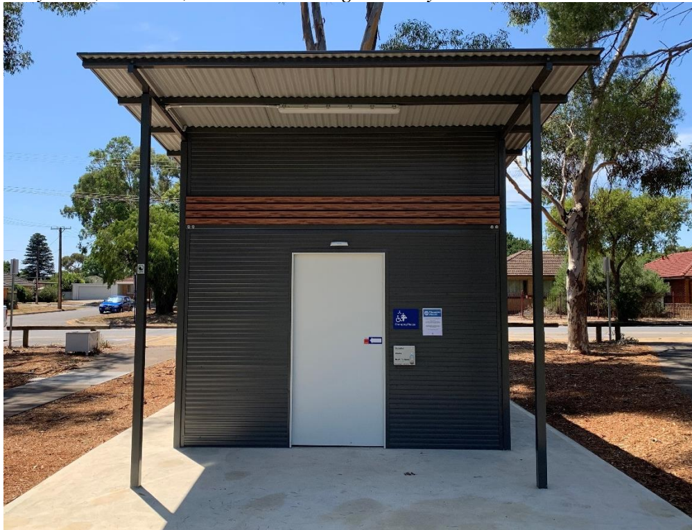
Unity Park, Pooraka, Accessible Change Facility
