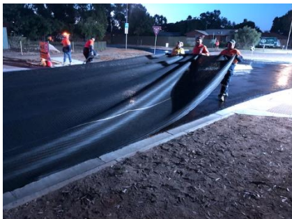
Nightworks on Lavender Road – Laying Ha-Telite as part of renewal treatment
