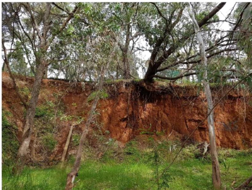
Photo 6: Failing banks undermining large established trees on top of batter. Which pose a risk to users of the reserve above and trail users below.
