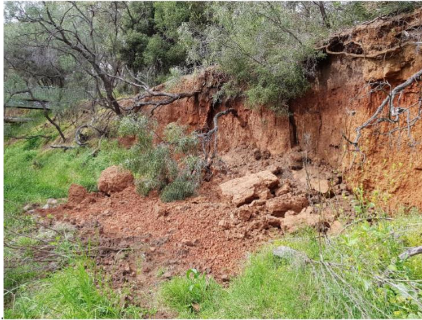
Photo 9: Recent embankment failure has also impacted on the vegetation. With losses being due to direct impact with the collapse of the bank and the dragging down of the vegetation that was established on the top of the bank.
