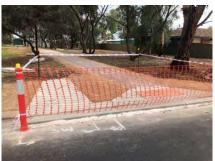
3.1 Base works are underway in preparation for the laying of asphalt paths at Springbank Waters, Burton, which continues the paths completed last financial year in the area.
