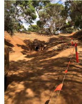
Dam Renewal Dam 24 Gulfview Heights
