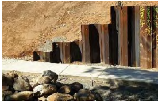
Underpass Main North Road, Pooraka
