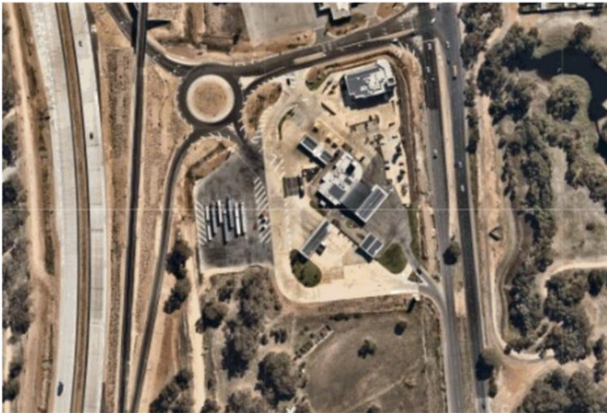
Figure 2: Updated image of site and locality showing completed works on the NEXY Source: Nearmap
