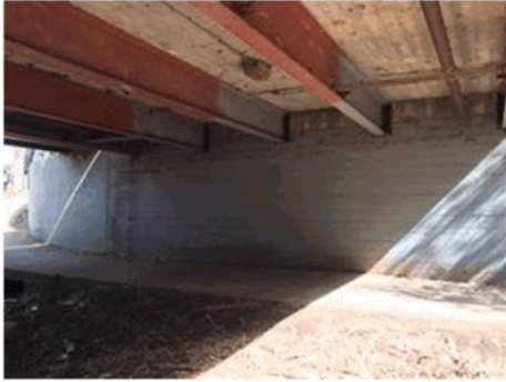
Pitman Park Underpass, 32 Gawler St, Salisbury
