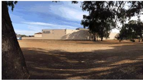
Paralowie Village Shopping Centre, 3-7 Liberator Drv, Paralowie
