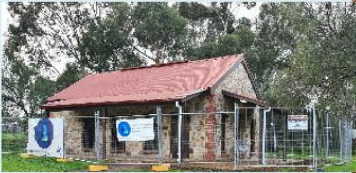
Water Wheel Museum, Salisbury Building Upgrade
