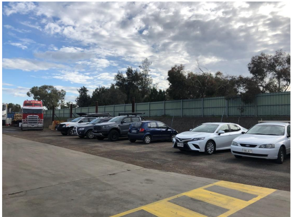
Photo 2. Looking north from the concrete hardstand toward the Council mound and fence, the new 6m barrier will be constructed inside of the mound and fence
