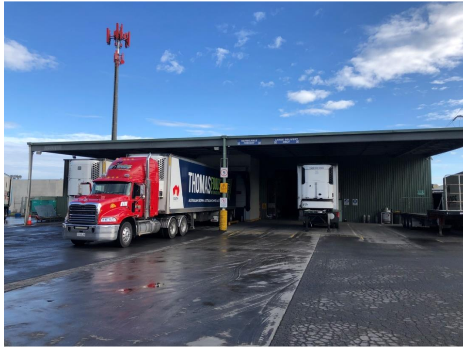
Photo 3. Looking north west from hardstand toward the coolroom, freezer and loading dock, Sonus have recommended a blade wall to enclose the side from the central column
