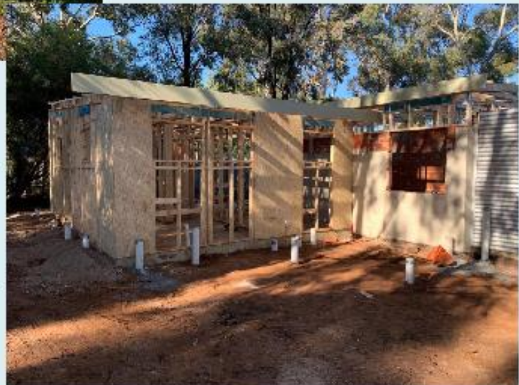
Pooraka Tennis Clubrooms Extension
