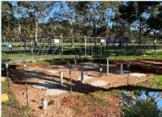
Unity Park, Pooraka, New Toilet Facilities
