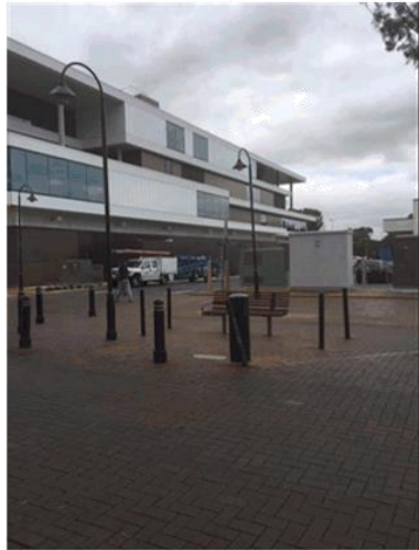
Figure 5-1 Bollards on John Street
