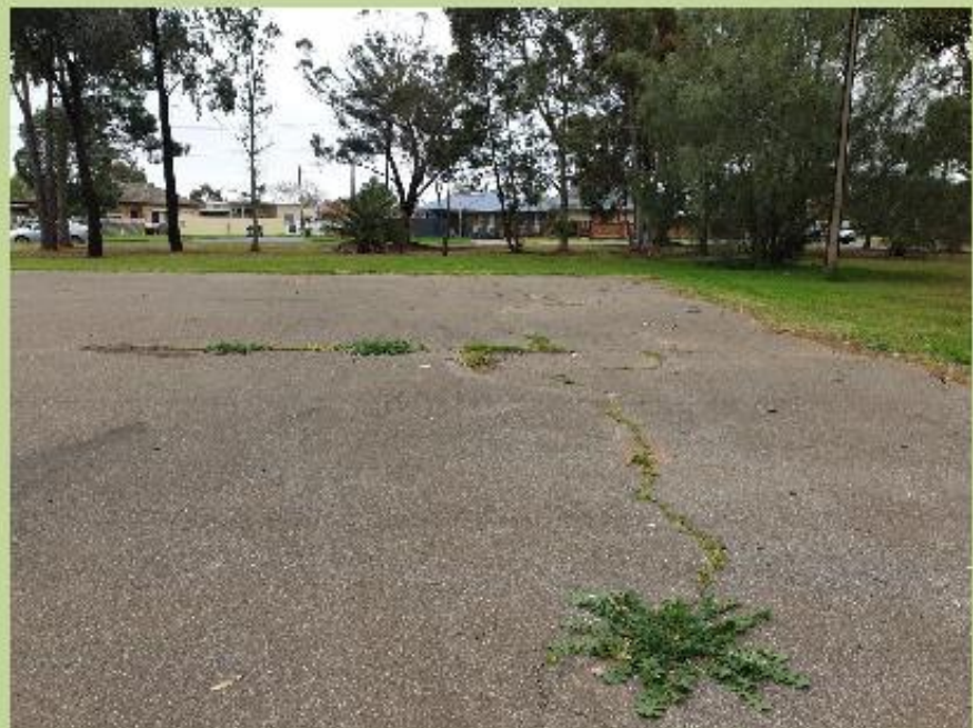
Salisbury Downs Oval Netball Courts Resurface
