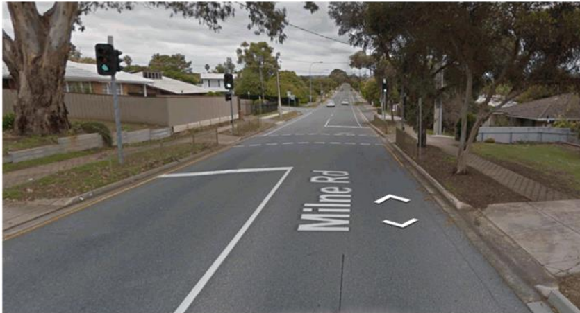
Figure 1: Pedestrian Actuated Crossing Installed on Milne Road near East Para Primary School
