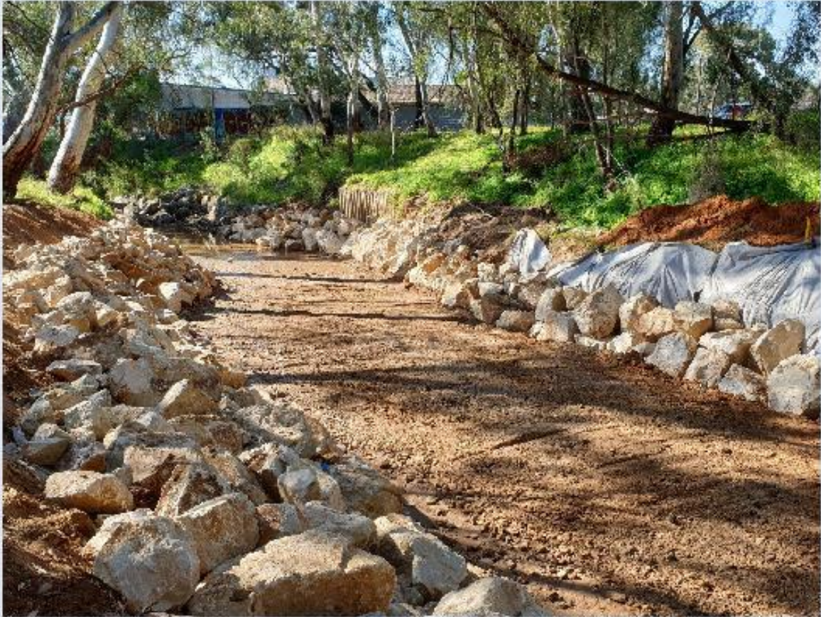
Dry Creek Watercourse and Erosion Works
