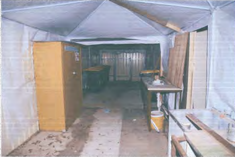
Area between the two buildings facing East showing the temporary cover provided by two gazebos.
