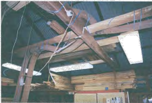
Storage of long timber in machine room.
