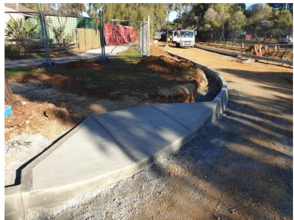
Halba Crescent, Paralowie, Major Flooding Mitigation, Work in Progress.
