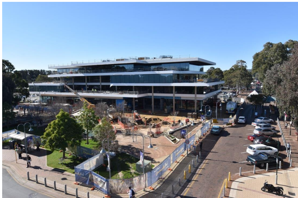
Photo 2: Soffit linings underway, all glazing installed, commencement of works to adjacent public spaces (Photo: 5 August 2019)
