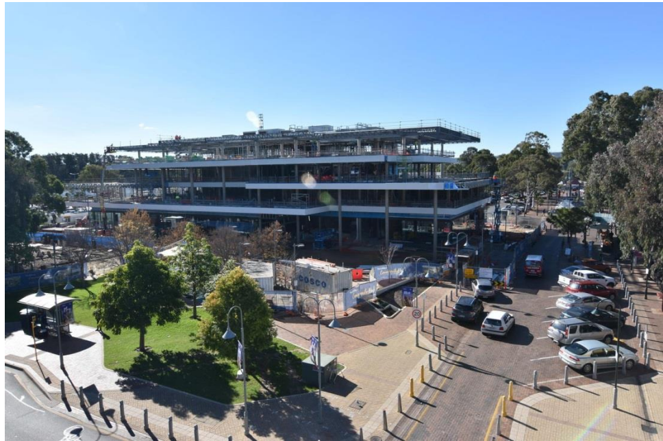
Photo 1: Roof Plant Slab upstands complete, Steel Roof Structure complete, Formwork stripping complete, Slab Edge fascia cladding and Ground Floor Glazing (Photo: 7 June 2019)
