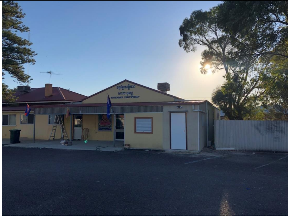
Photo 4. Looking west from car park toward the Meeting Hall
