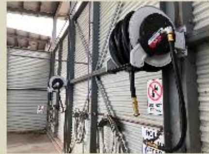
Renewal Works, Wash Down Bay, Operations Centre
