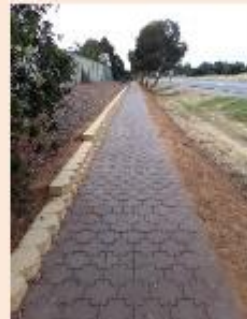
Elder Smith Road, Mawson Lakes, New Footpath
