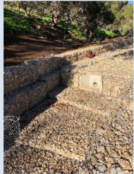
Coomurra Gully Reserve, Salisbury Heights, Major Flood Mitigation Works
