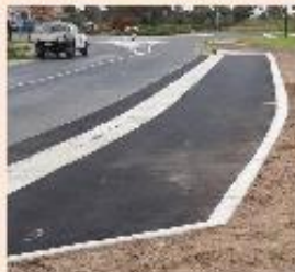
New indented parking bays, Springbank Waters, Burton
