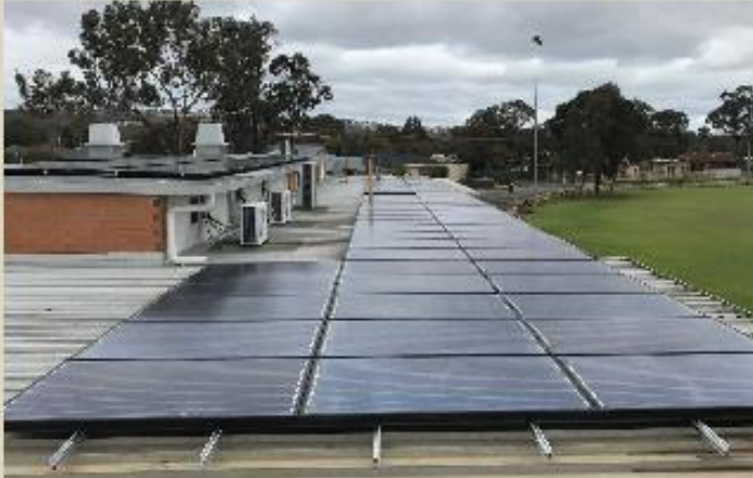
New Solar Panels, Brahma Lodge Oval
