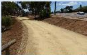
New dam access track was constructed in Para Hills
