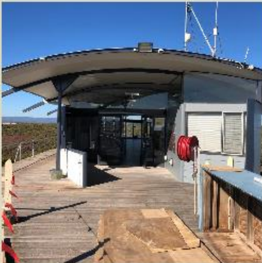
St Kilda Interpretive Centre, Building Renewal Works in Construction
