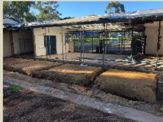
Salisbury Recreation Precinct, Salisbury North, Building Upgrade, Work in progress
