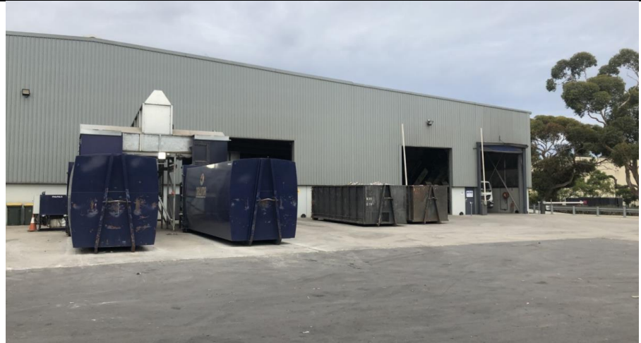
Photo 2. Looking south-west from rear hardstand toward existing building and external compaction containers and glass bins
