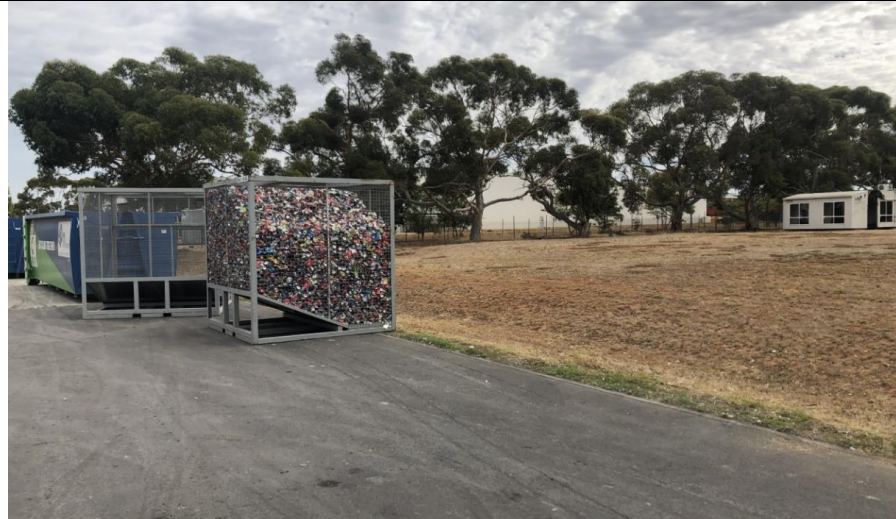
Photo 6. Looking north-west from rear hardstand toward side boundary fence and Tugger Way
