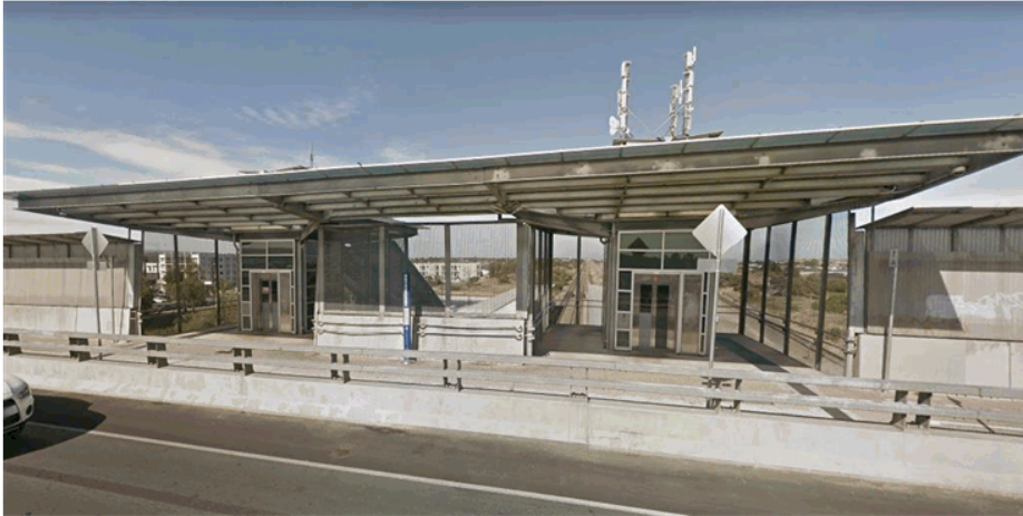
Figure C.10: Mawson Lakes Interchange Bridge on Elder Smith Road
