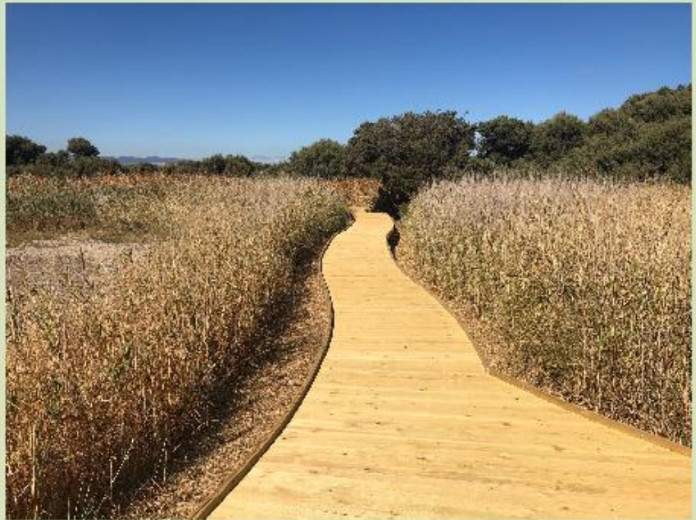
Approximately 82 metres of boardwalk was replaced within Greenfields Wetlands
