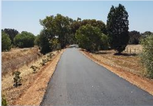
Parafield Bituminous Path Renewal
