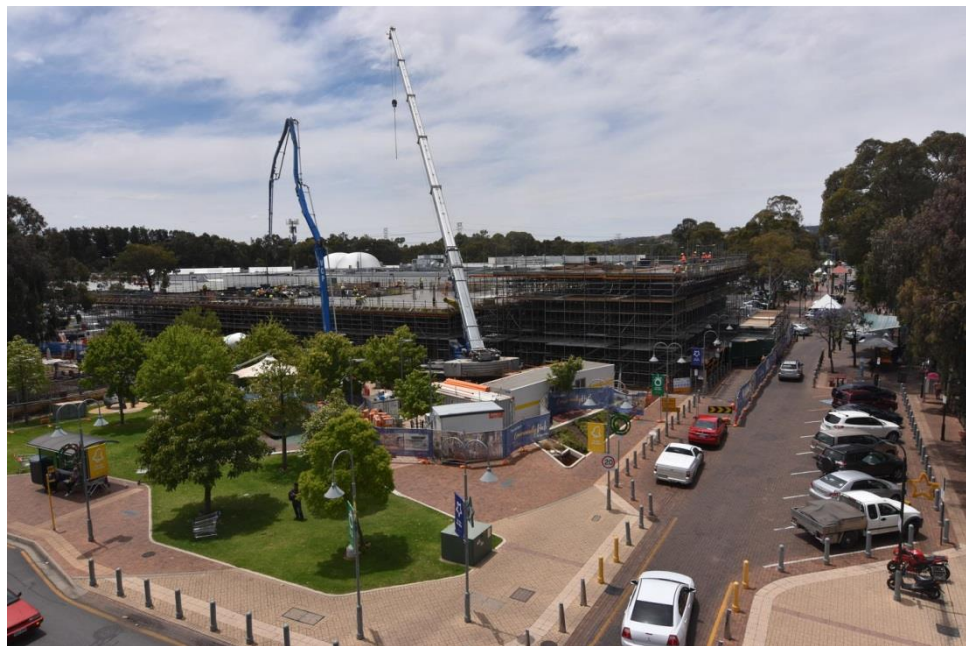
Photo 1: Level 1 Slab Pour, Level 2 Formwork John Street (Photo: 27 November 2018)
