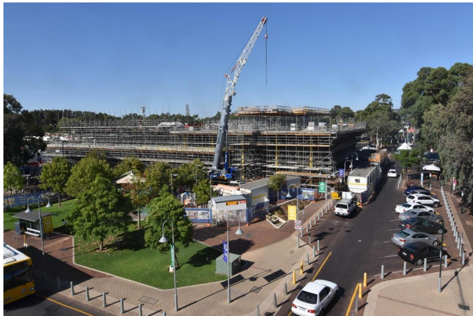
Photo 2: Level 3 Formwork John Street (Photo: 21 January 2019)
