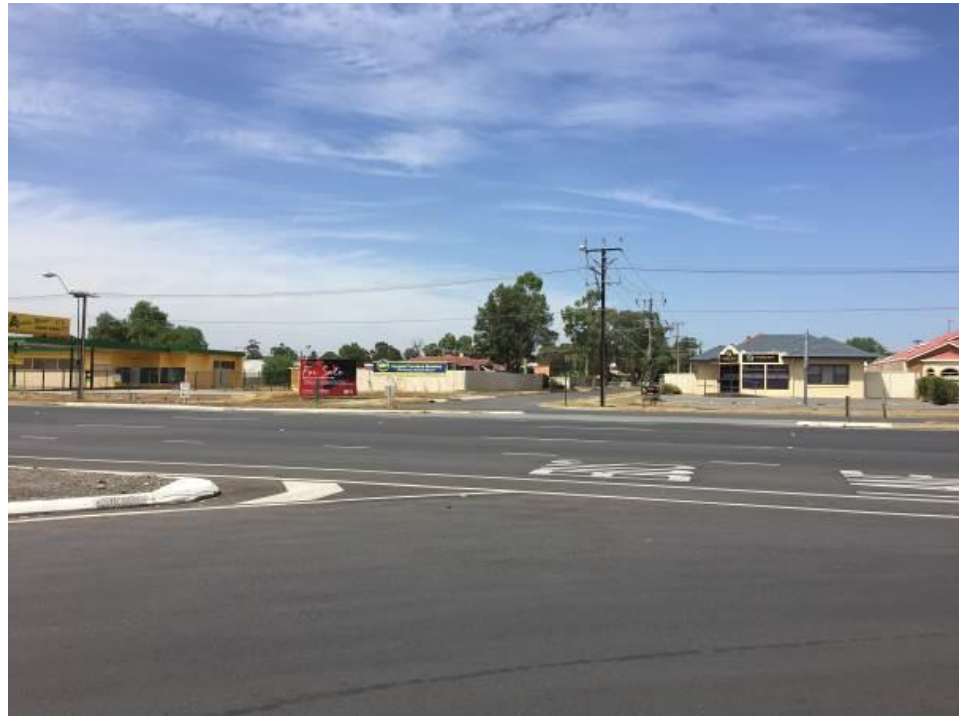
Photo 7. Looking east from Market Lane towards the subject site (right hand side) on the southern side of Royal Avenue and the site located in the Commercial Zone (left hand side) located on the northern side of Royal Avenue)
