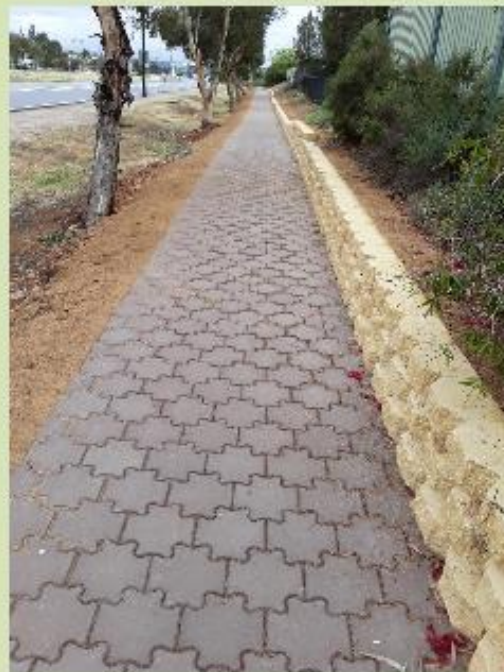
Elder Smith Road, Mawson Lakes Council Funded New Footpath Program
