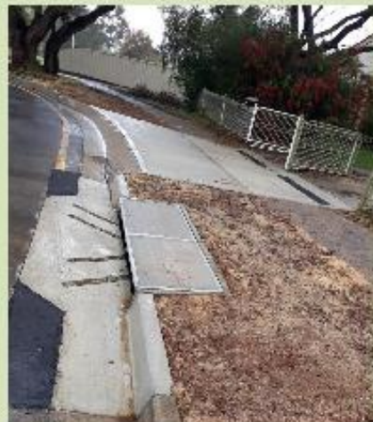
Nelson Road, Local Flooding Program
