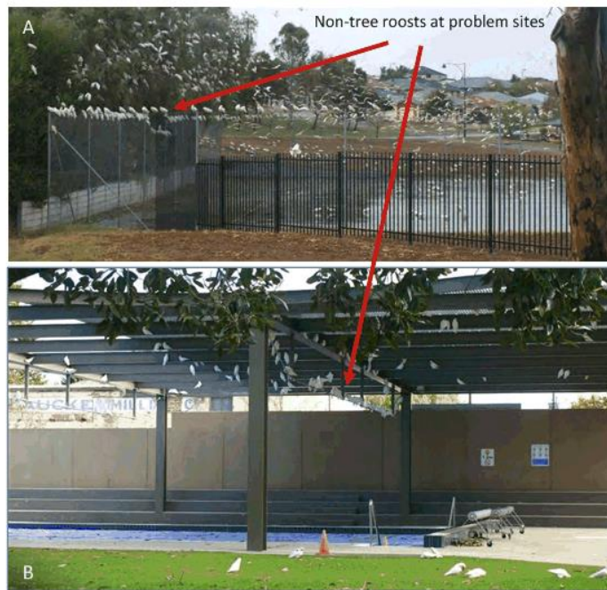
Photo panel 10 Non-tree roosts at problem sites
