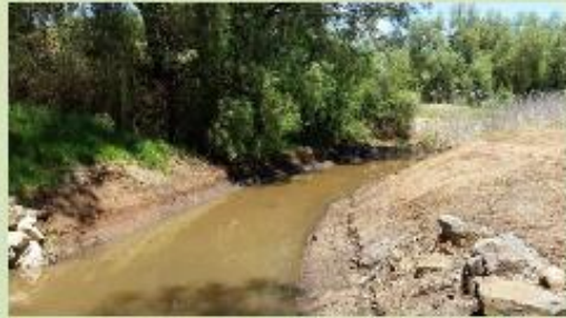
Little Para Erosion Control Works Watercourse Management Works
