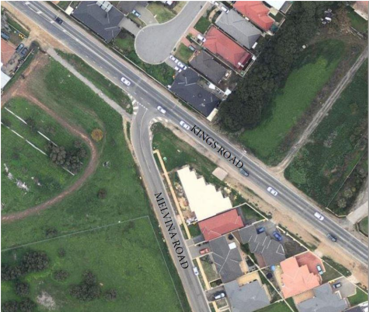
Item 2.7.3 - Attachment 1 - Kings Road and Melvina Road - Original intersection layout (aerial image)
