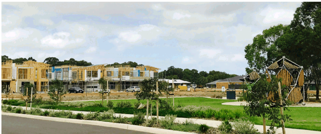
Jewel Living under construction, visible from the project entry park.
