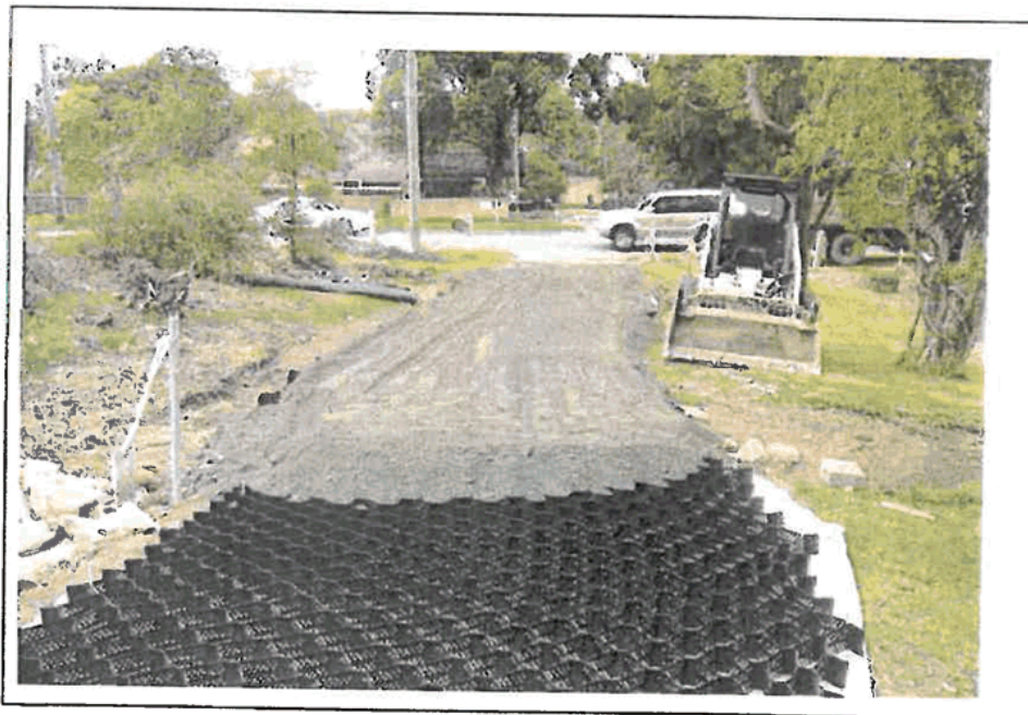
Image 8: The use of Eco Cell above the natural soil with 20mm gravel to allow yearly access; this is a viable option for the palms to allow reasonable access under the False Date Palms without causing structural root damage.
