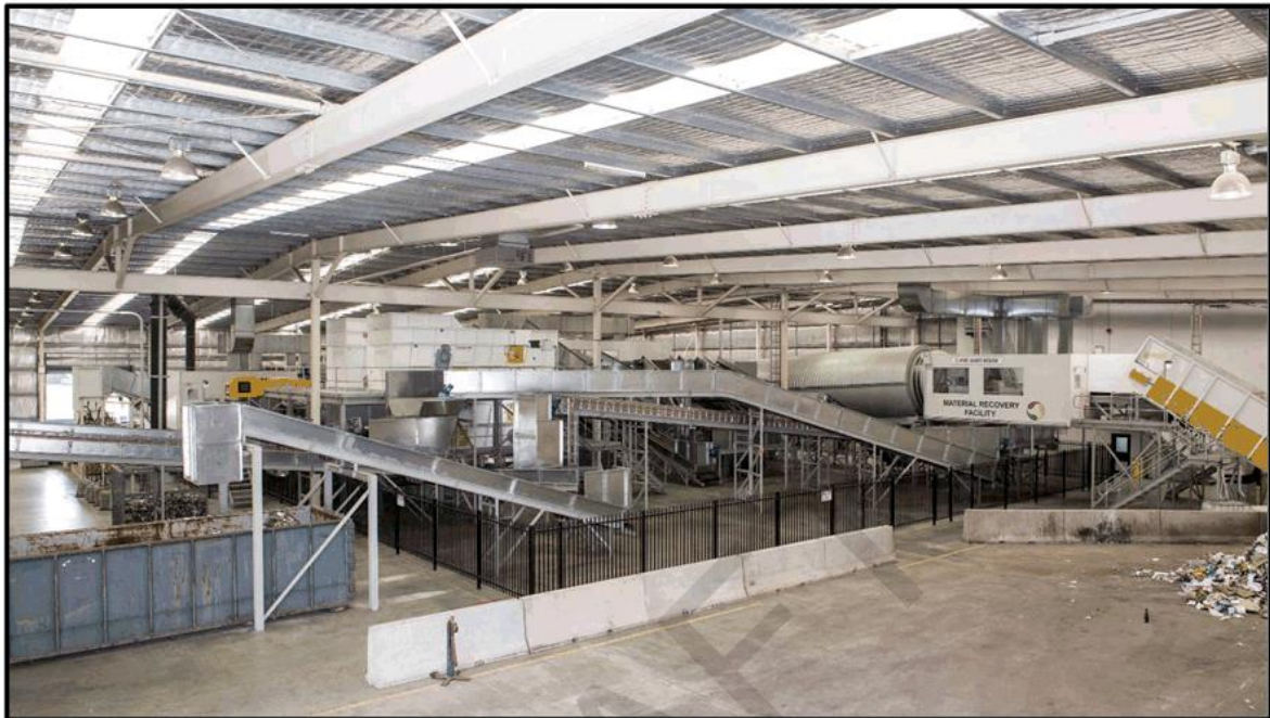
Image: Operational Material Recovery Facility (MRF)
