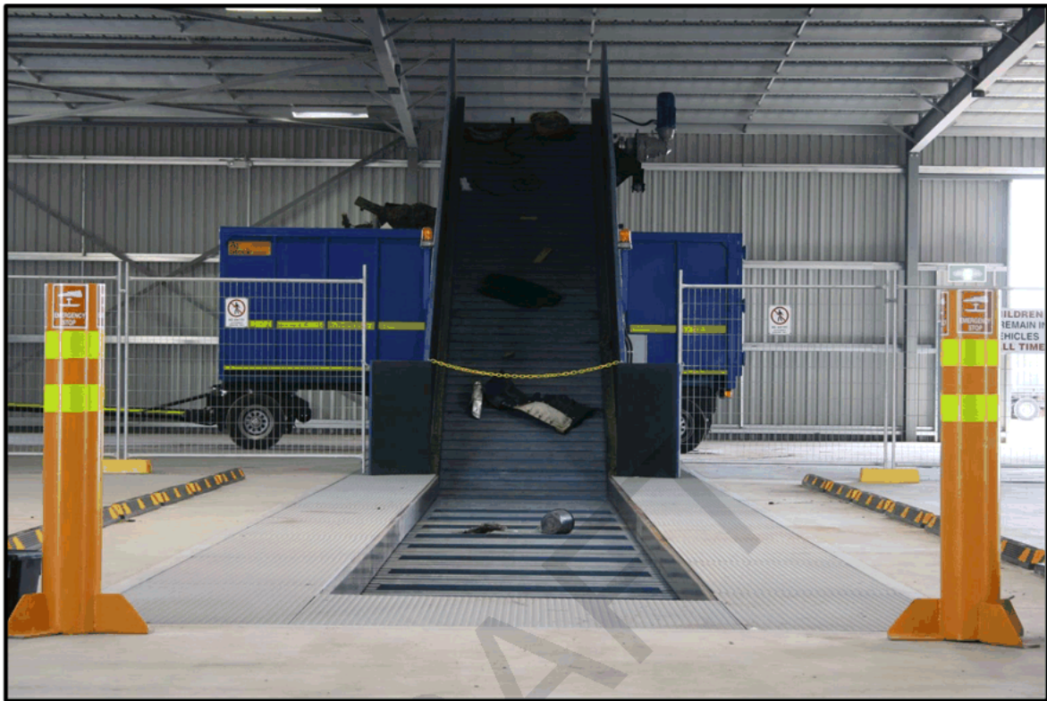
Image: Inside NAWMA's Edinburgh North Public Transfer Station
