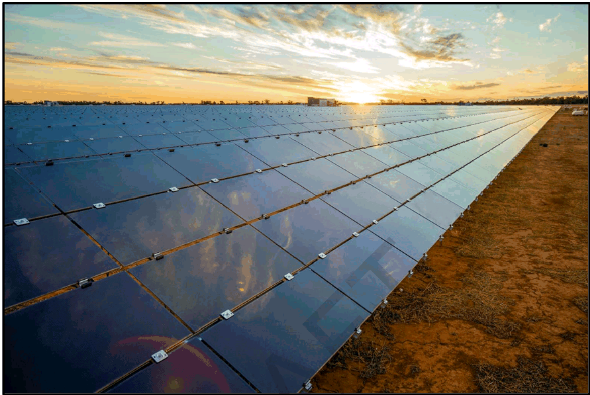
Image: Solar thermal energy at Uleybury Landfill
