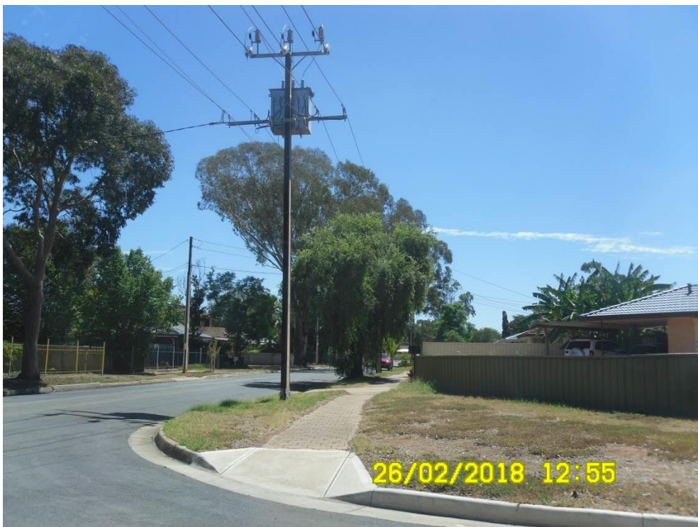
Photo 2: Looking north from the intersection of Malcolm Street & Margaret Street
