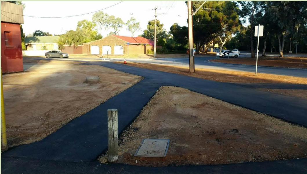
Cross Keys / Frost Road, Bicycle Network Improvement
