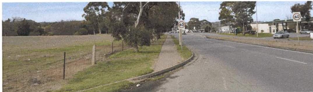
PHOTOGRAPH 03: TERMINATION OF THE FOOTPATH ON KINGS ROAD
