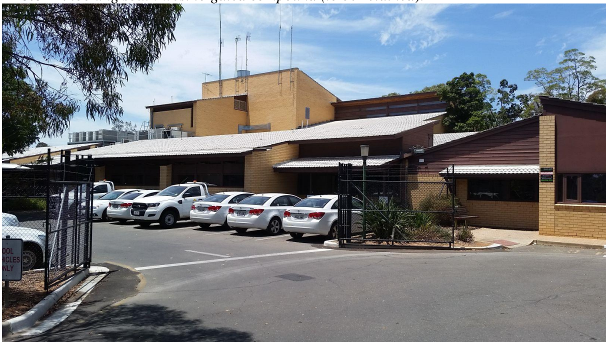
Photo 11: looking south west to gated compound (to be retained).
