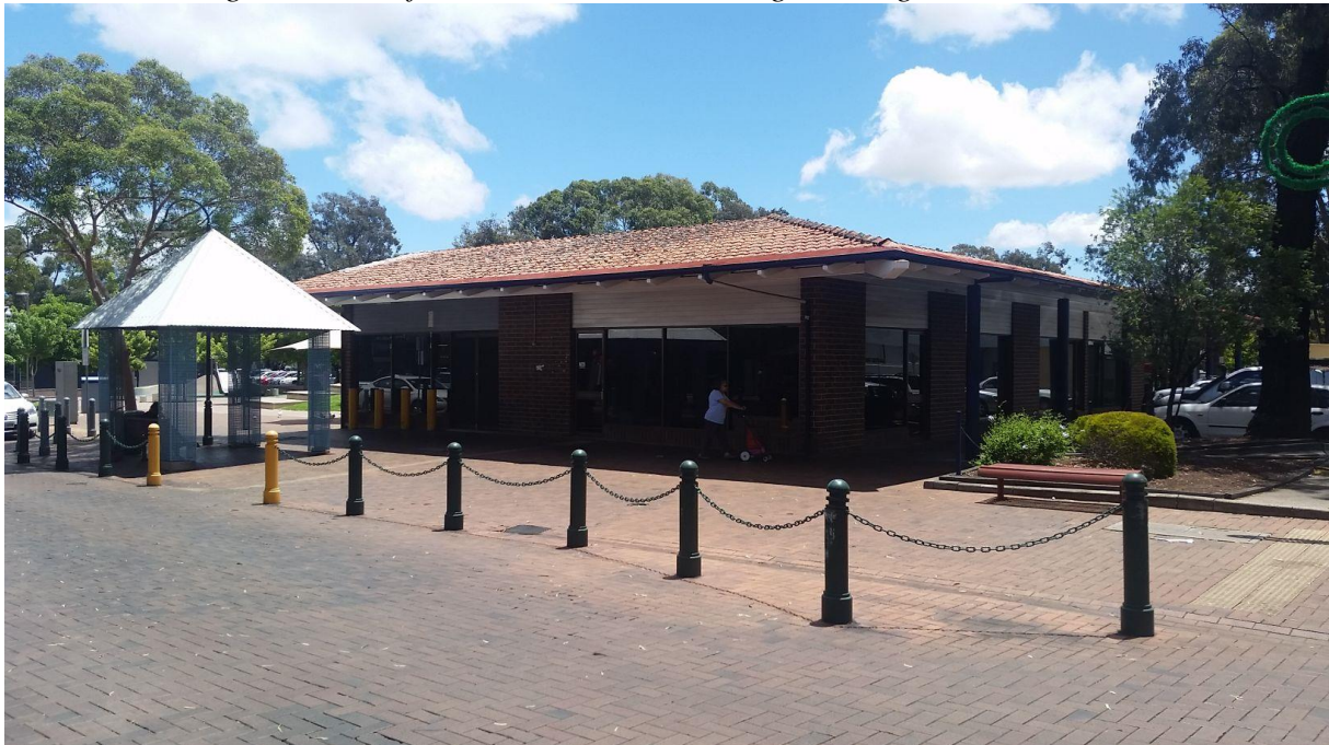
Photo 5: looking north-west from John Street – existing building to be demolished.
