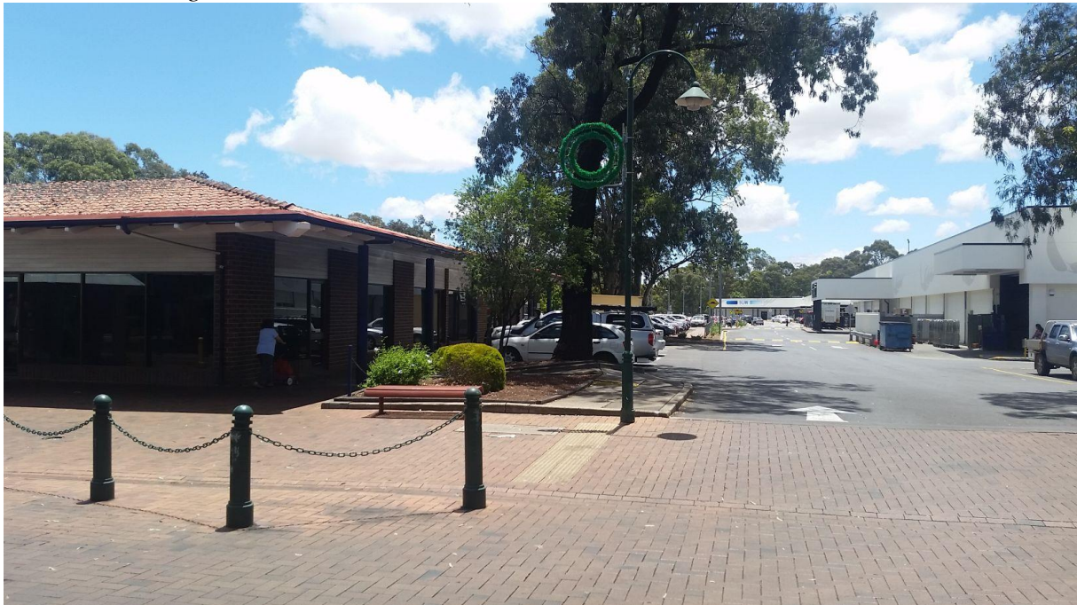
Photo 6: looking north from John Street – existing building to be demolished on left / Parabanks on right.
