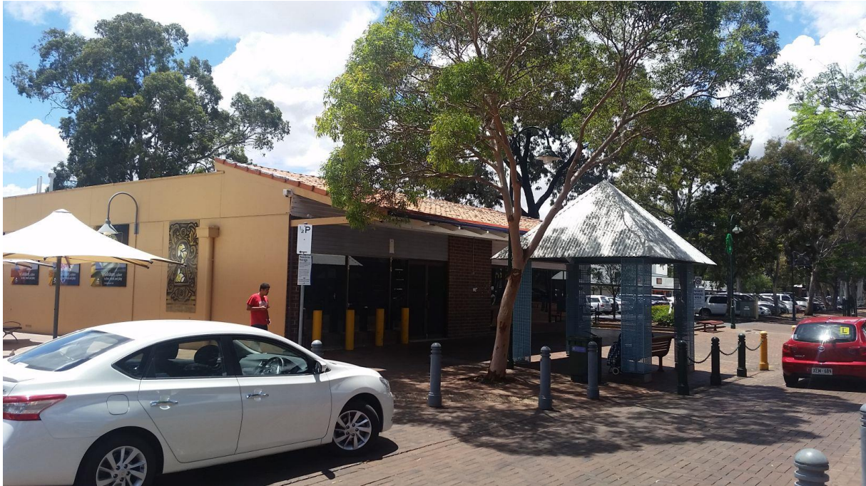
Photo 4: looking north-east on John Street – existing building to be demolished (and affected street tree).
