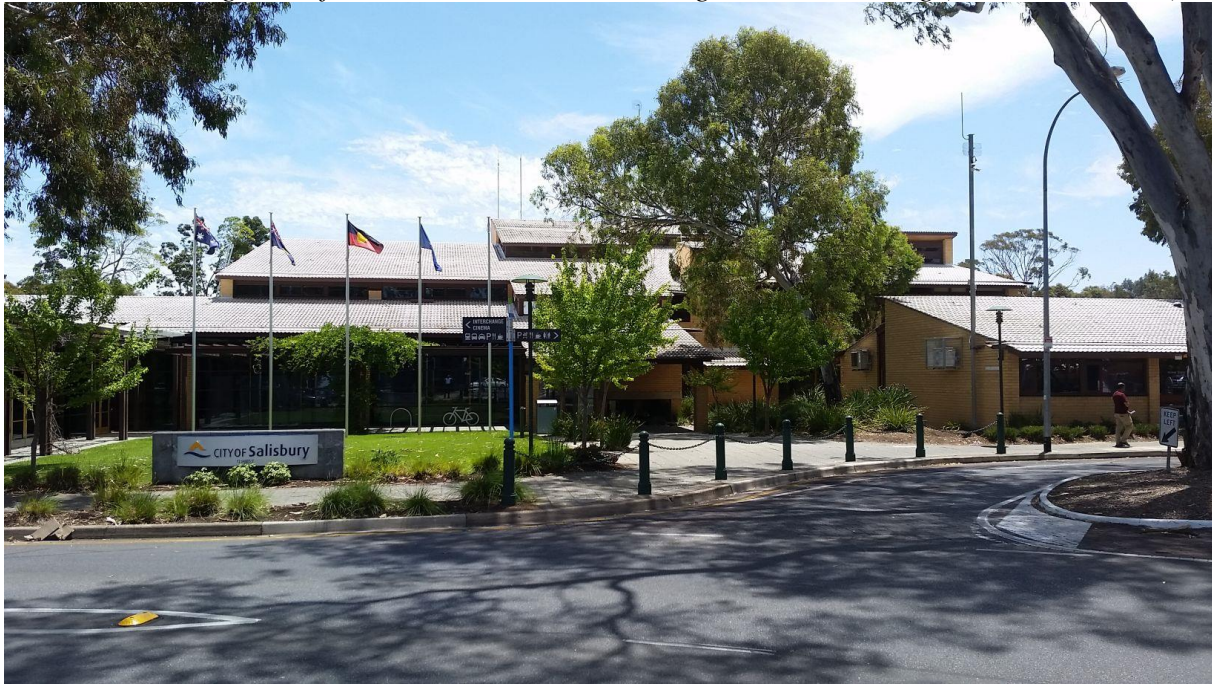
Photo 10: looking north from Church Street to existing Council building (to be demolished).
