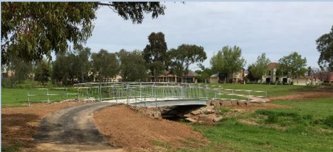
Bridge Renewal, adjacent Victoria Court
