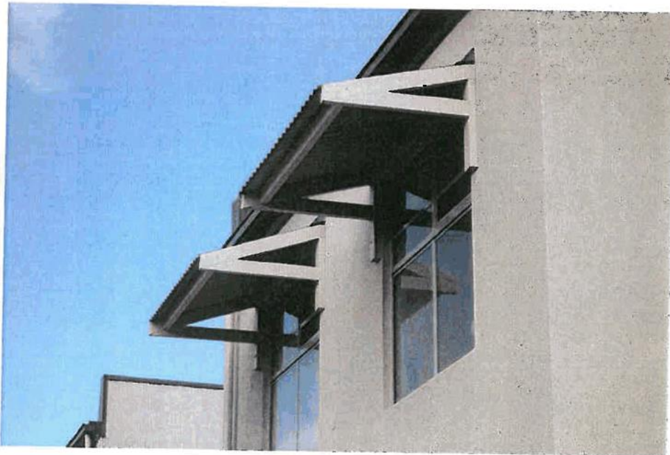
Above and below - Alternative upper level window opening design for varied upper level north elevation for units 1-5 allowing for lower panel to be obscure glazing, with upper portion restricted opening. Example from approved Distinctive Homes development, Joseph St, Salisbury (final detail of glazed panel proportions may not match this exactly).
