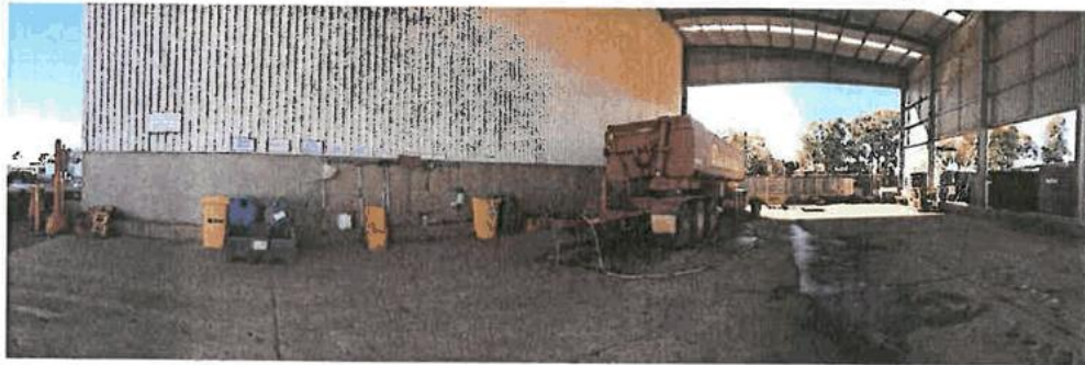
Overview of wash pad
