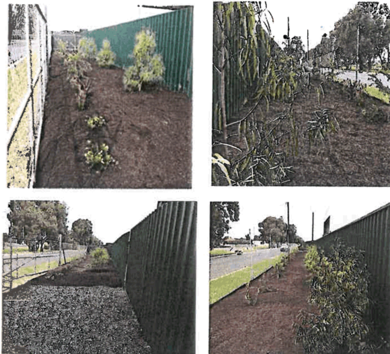
Figure 1 Landscaping at Helps Road completed on the 6 th of October 2017
