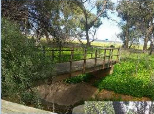
Bridge Removal, Parafield
