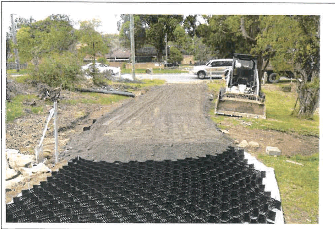
Image 8: The use of Eco Cell above the natural soil with 20mm gravel to allow yearly access; this is a viable option for the palms to allow reasonable access under the False Date Palms without causing structural root damage.
