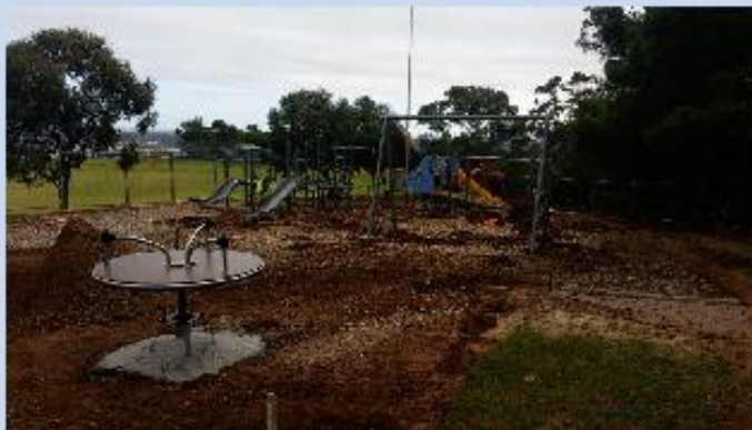
Para Hills Oval Playground Renewal
