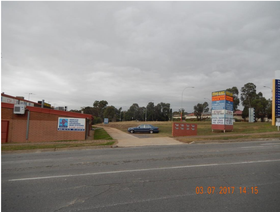
Photo 2: Standing on the southern side of Research Road looking north toward the building, single-width cross-over and signage. This is the eastern portion of the land.
