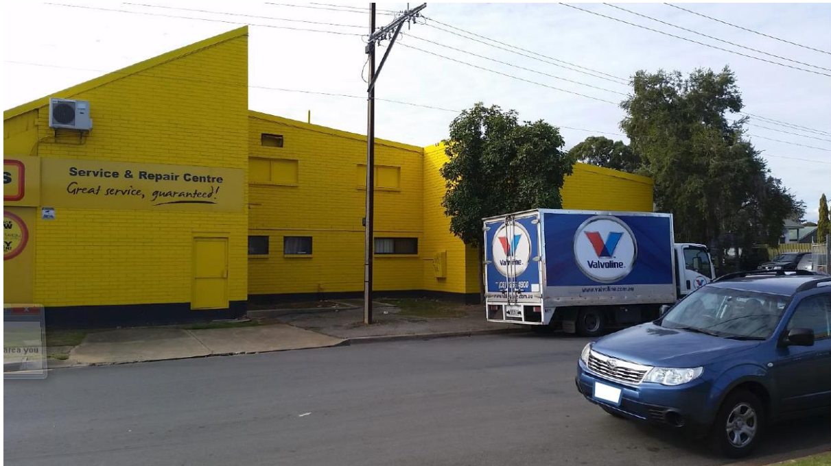
Photo 5: Looking north-east across Fleet Street from the front of the subject site
